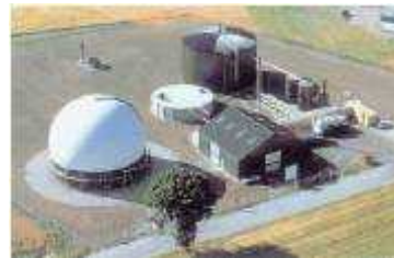
JFE bigadan biogas system
