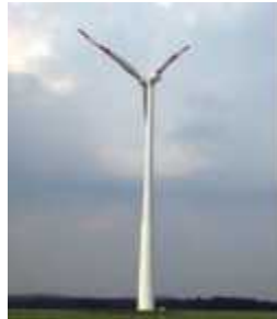
Ebara wind generator
