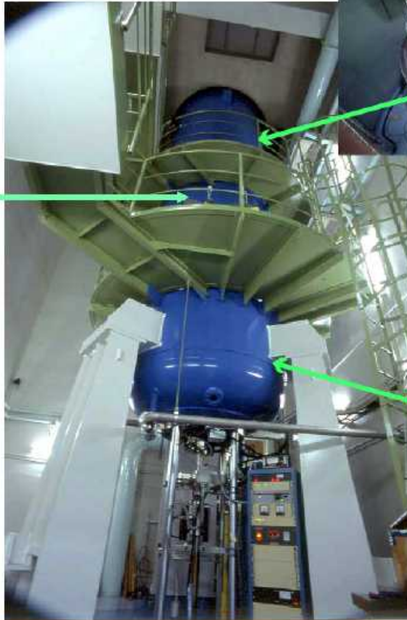
Looking up the Accelerator Tank
